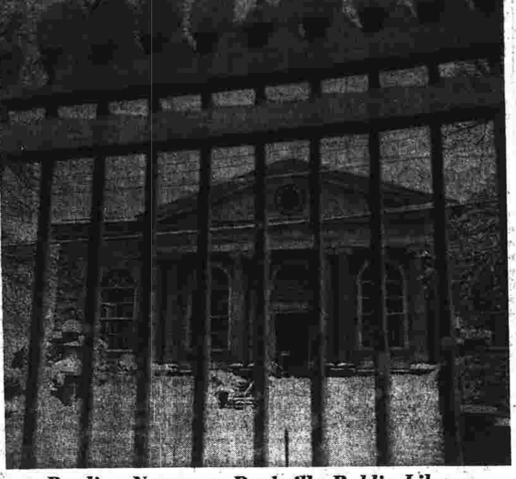
Battling Nature at Rockville Public Library George Gregus, the custodian of the Rockville Public Library, barely visible through the iron fence in front of Rockville General Hospital, begins to clear the broad steps that front the library of last night's foot-deep snow fall. Before he is done, Gregus will clear the steps for their entire width—not a job, unfortunately, that can be done with a snow blower. (Herald photo by Bateman.)
